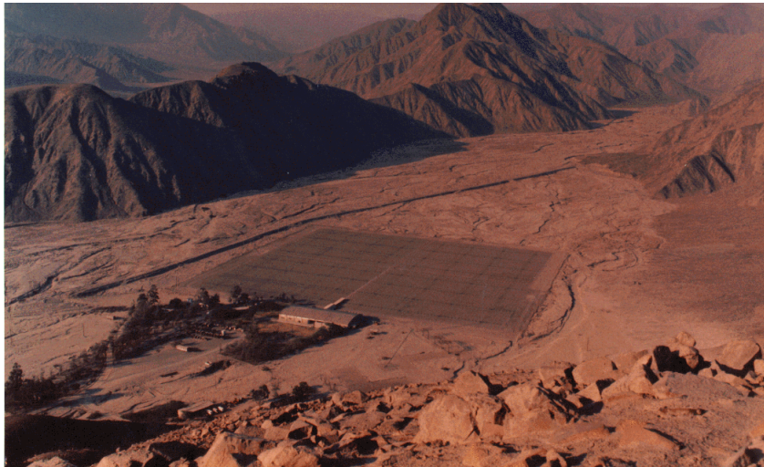
49.92 MHz incoherent scatter radar at the Peru Observatory The radar has an array of 18,432 half-wave dipoles !!
