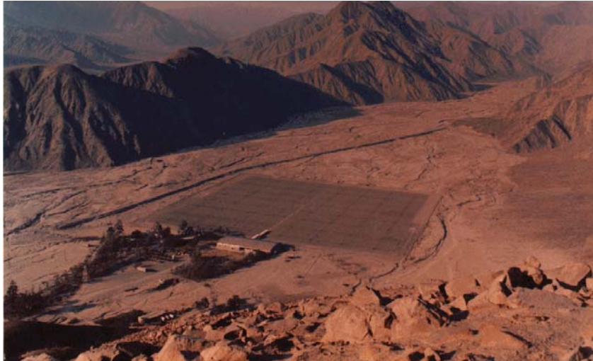
49.92 MHz incoherent scatter radar at the Jicamarca Observatory The radar has an array of 18,432 half-wave dipoles !!
